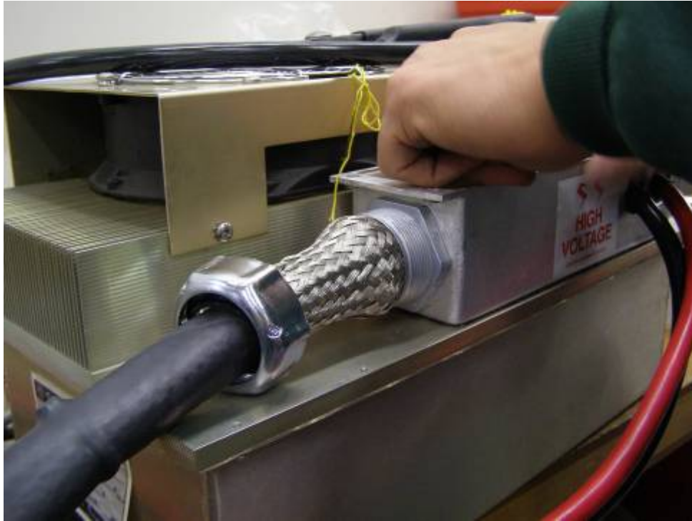
Figure 7. Shows AC motor cable inserted into entrance fitting with 360 degree connection of the cable shield to the inside wall of fitting.
